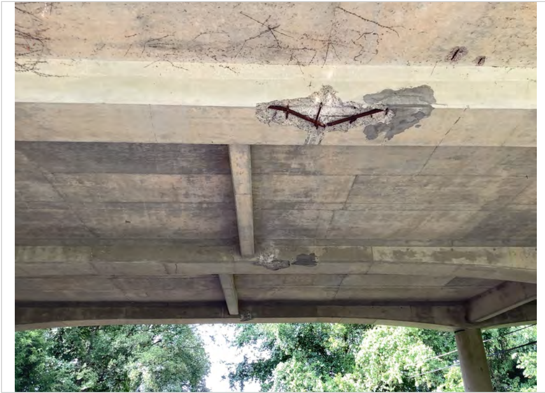
Collision damage to beams in span #2
