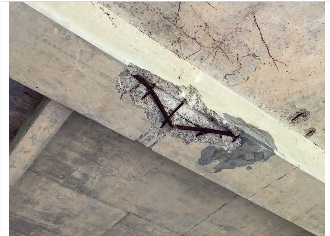
Broken steel reinforcing in beam "A" in span #2
