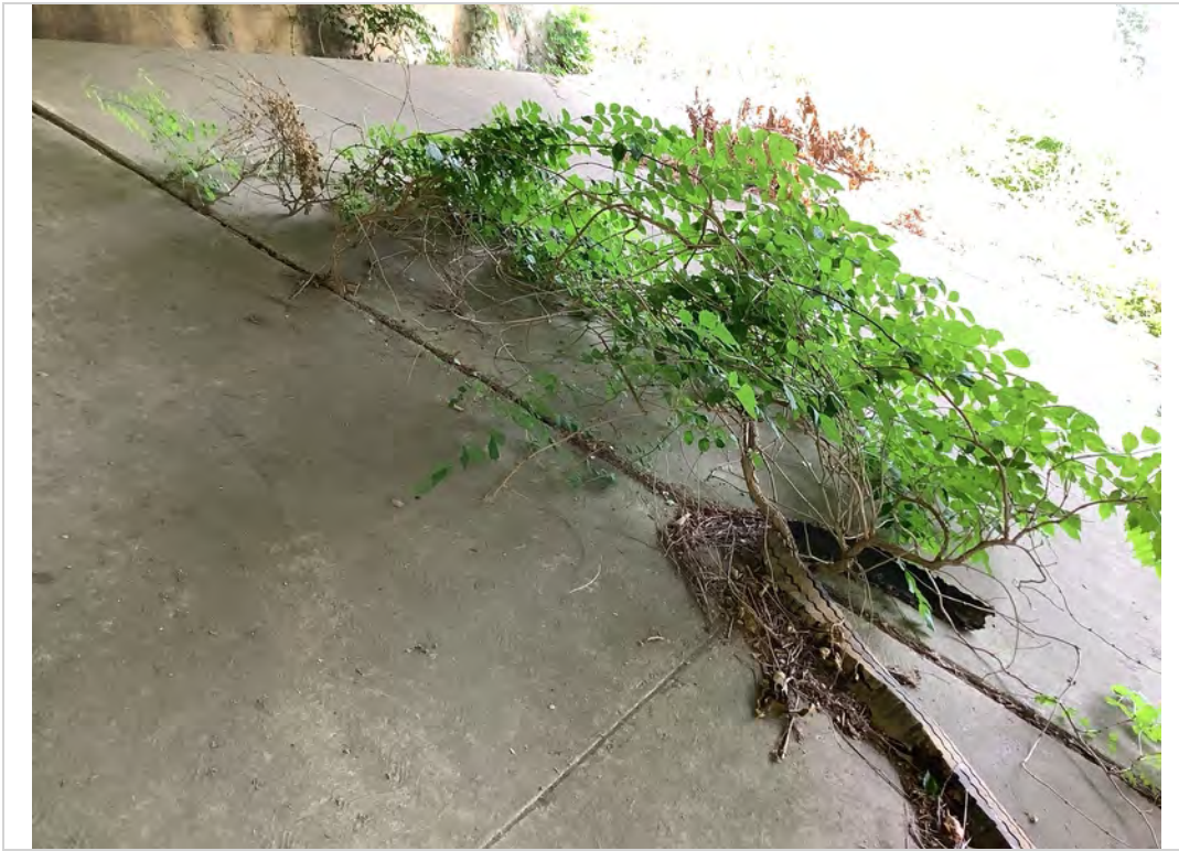
Vegetation growth between cracks in slope paving
