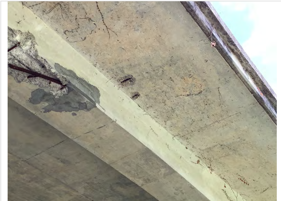
Typical spall in overhang
